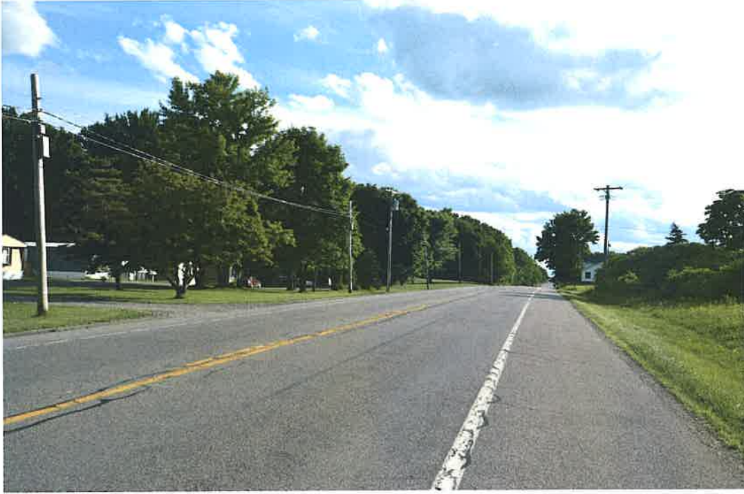
Route 33 at Dublin Road looking Southwestly.
