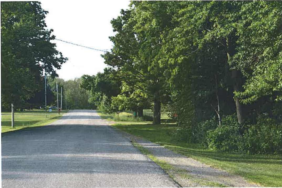
School Road at LeRoy Town line looking Northerly.
