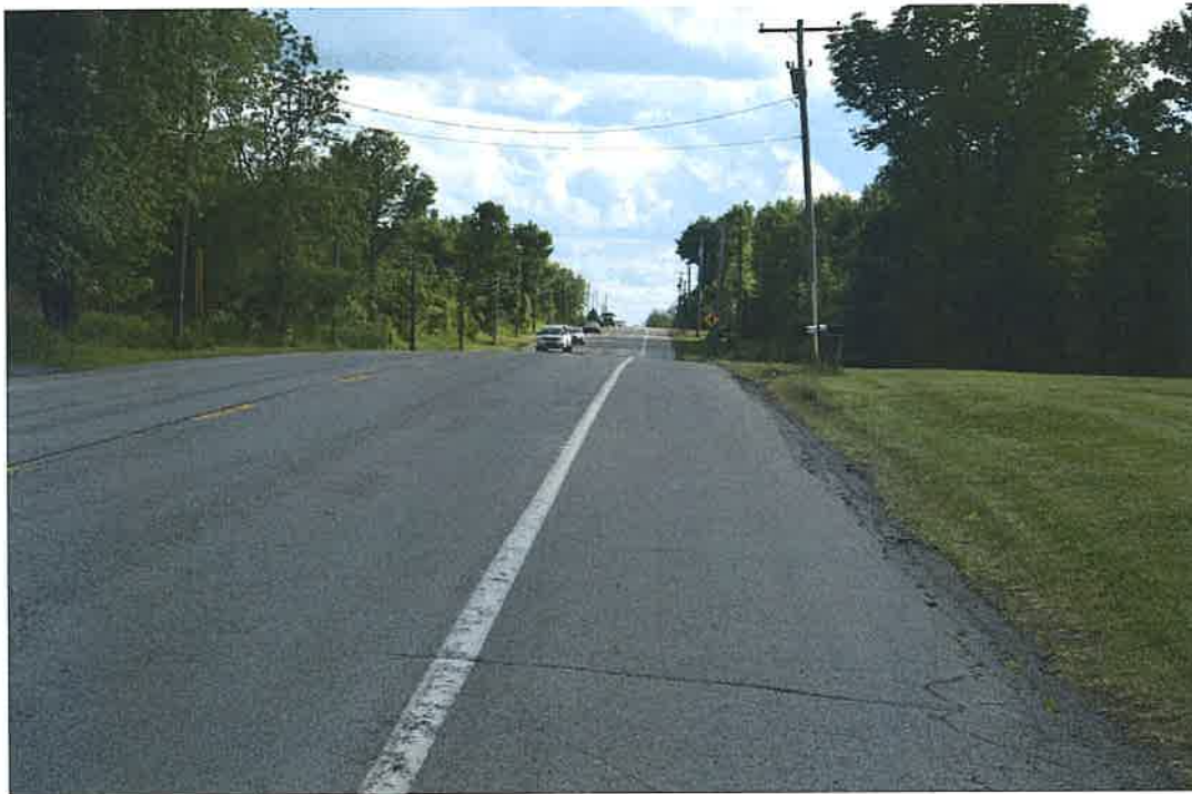
Route 33 at Jerico Road looking Southwesterly.
