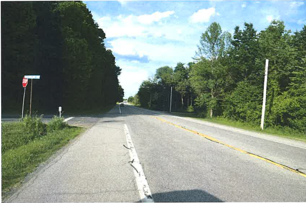
Route 33 at Dublin Road looking Northeasterly.
